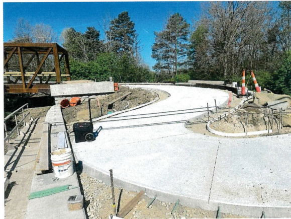
Switchback being installed on the west-end near bridge
