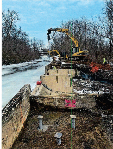
Ohio & Erie Canal spillway still intact with helical piers for new bridge being installed.
