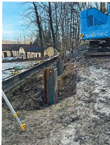
Crane installing metal supports for retaining wall sections.
