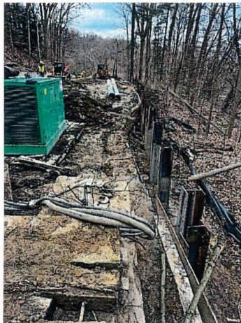
Old retaining wall leaning up against the new metal supports of new retaining wall.
