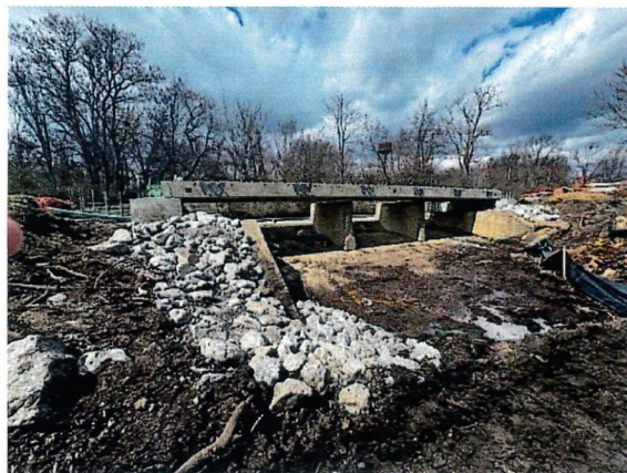
Ohio & Erie Canal spillway still intact with bridge beams installed.
