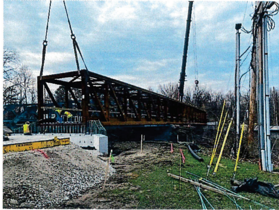
Bridge over CSX Railroad Corridor being put in place.
