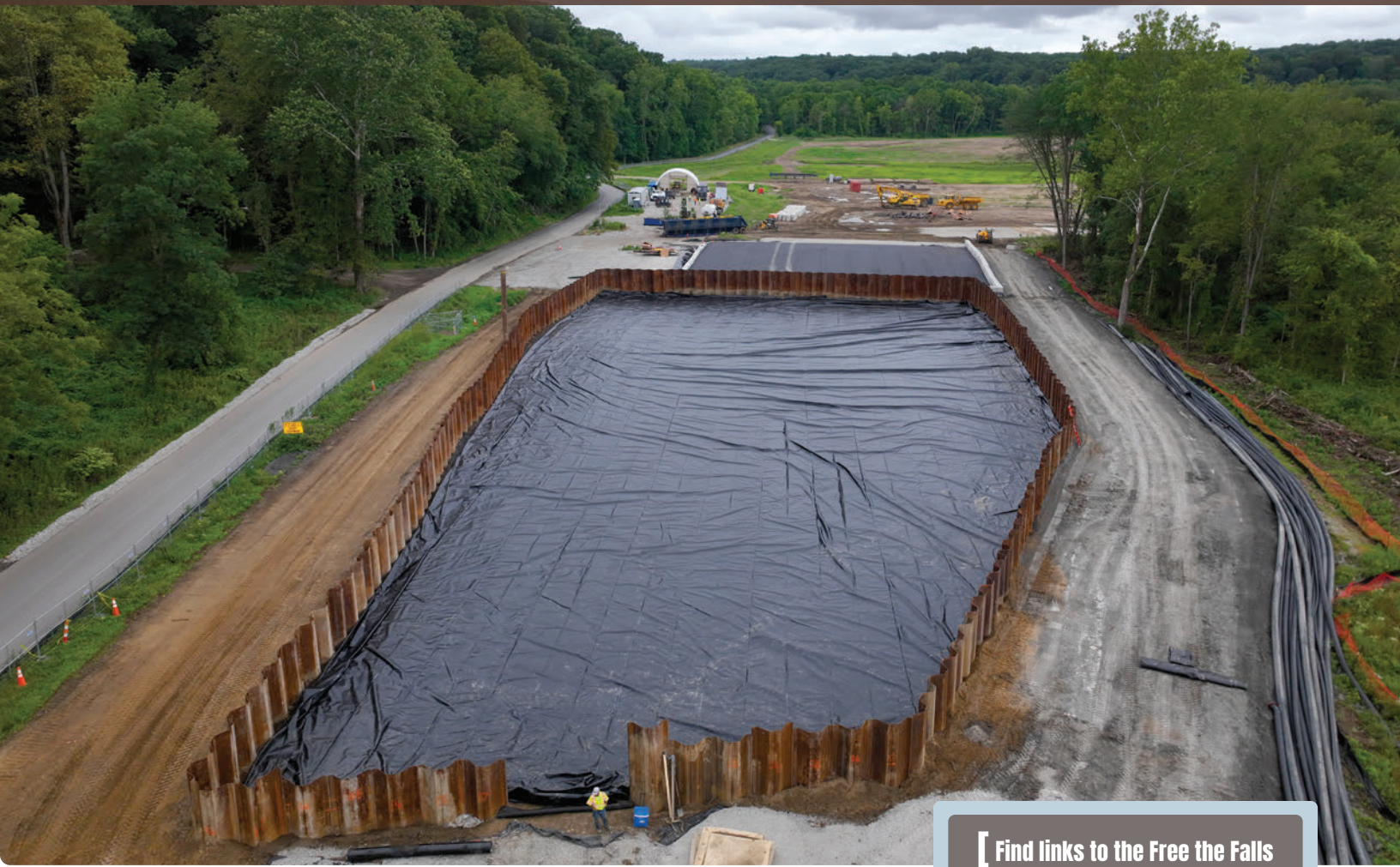
An aerial view of the sediment surge basin, the first step for sediment before it is processed for final placement. (August 2025)
