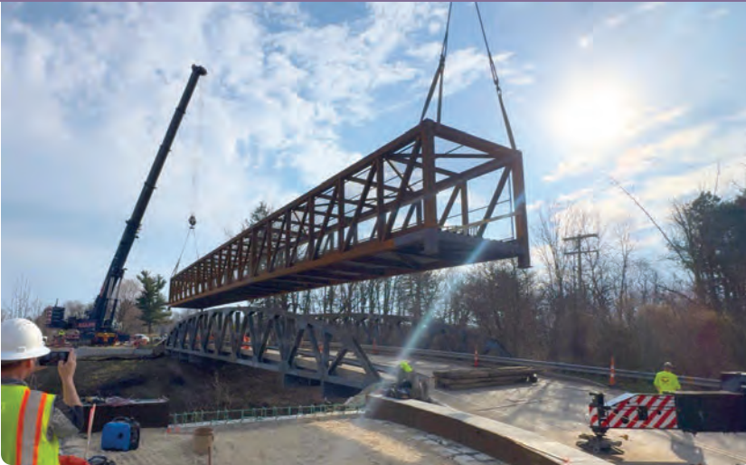
Cranes lift a metal pedestrian bridge placed as part of the Middlebury Road connector project.
