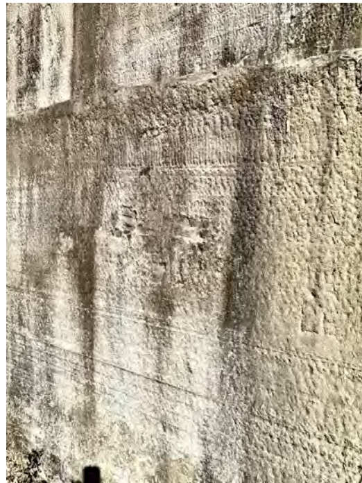
Note the tool marks on the face of the quarry wall
