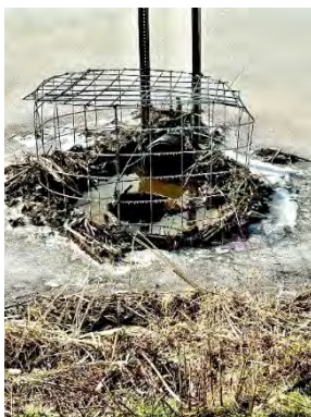
The spillway (called a glory hole spillway at Sylvan Pond. The pipe is a distance from the dam, minimizing flowing water near the dam preventing erosion. The pipe goes down and under the dam, discharging downstream. There is an overflow spillway at the side of the dam to prevent floodwaters from overtopping and eroding the dam.
