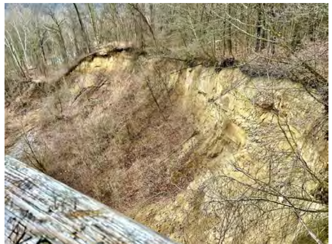
The slope face to the west of the overlook platform is composed of outwash. Note this slope is easily erodible.
