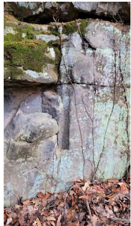
Drill hole used to place explosives
