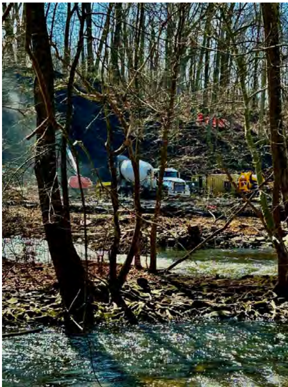
Work being conducted (March 2024) at the Chuckery Area. Gunnite was being applied to the shale rock face for slope stability. Gunnite is basically a thin concrete applied with a hose.
