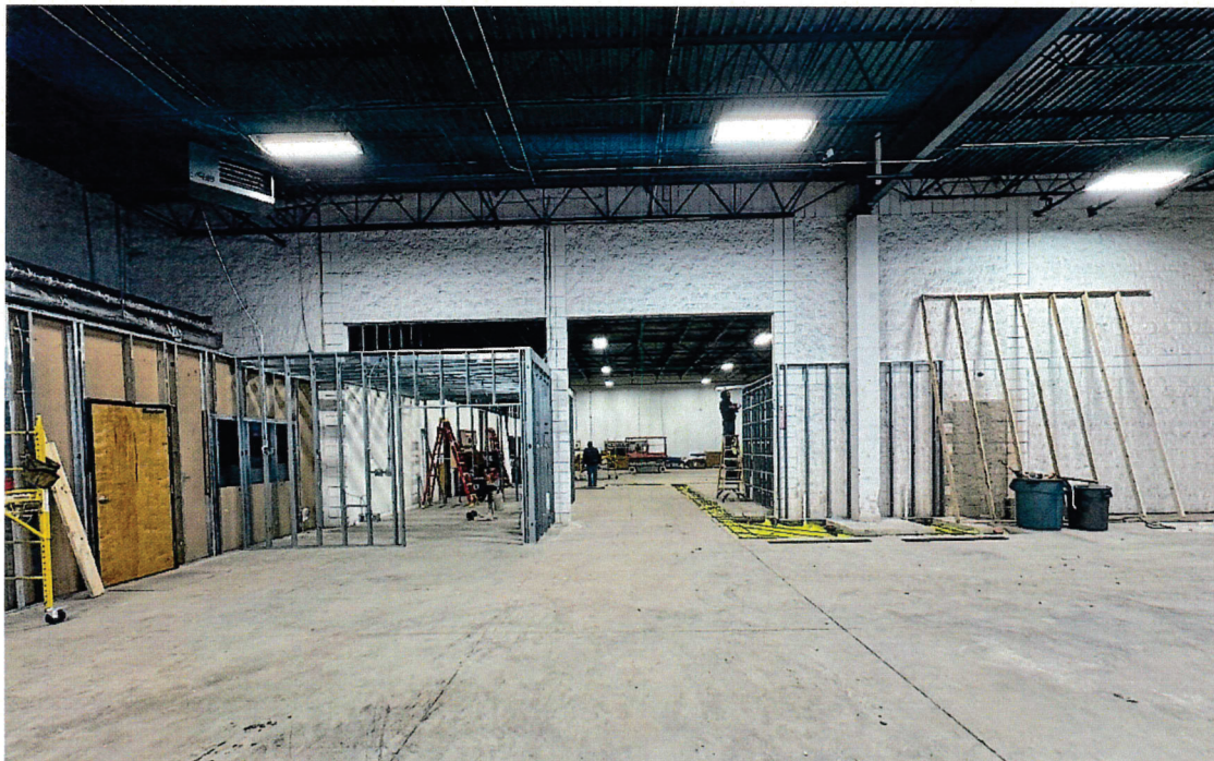
Framing walls with additional drainage on floor ready to pour concrete.
