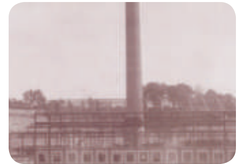
In 1911, construction of the Northern Ohio Traction & Light Power Plant on the Cuyahoga River, north of the dam, contributed to the end of High Bridge Glens.
